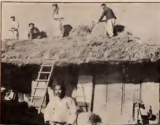
Koreans did not stand idle when war burned their homes. Here villagers pitch in, thatch new roof with rice straw.
